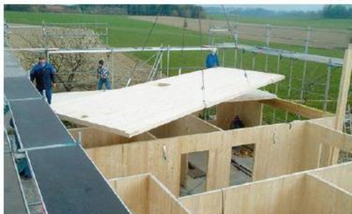
Figure 5 : Panneau massif contrecollé ou cross laminated timber (CLT) – source FCBA
